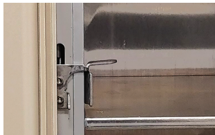
Easy release handle to open master gate
